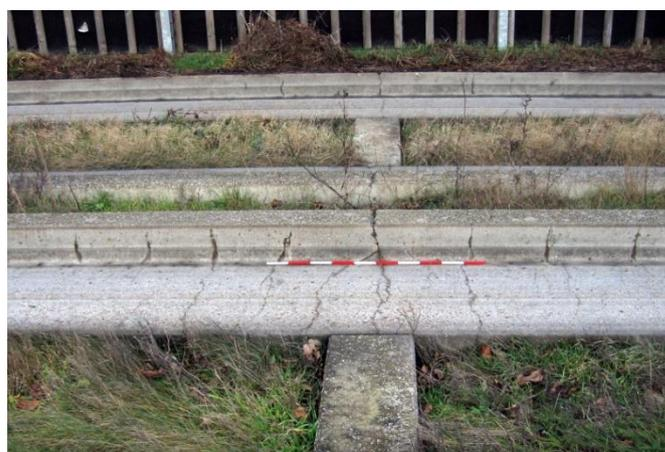
An earlier consultants' report does not appear to get to the root-cause of the problems regarding cracking and misalignment of the concrete beams that have occurred during the first five years of its projected 40 year lifespan.
